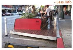
The design of a parklet should not inhibit the adequate drainage of stormwater runoff. Small channels between the base and the platform facilitate drainage.
