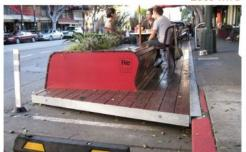
The design of a parklet should not inhibit the adequate drainage of stormwater runoff. Small channels between the base and the platform facilitate drainage.
