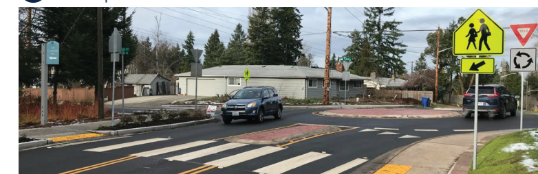
2 Paved Splitter Island at Roundabout to Accommodate Truck/ Bus Access
