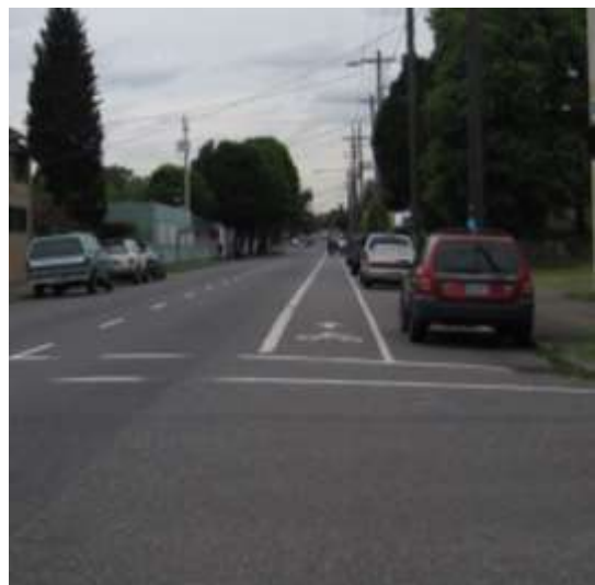
[53] Example of standard on-street bike lane (Source: DKS)
