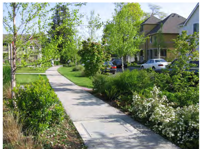
Porous paving on sidewalk
