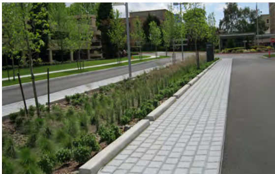
Swale in roadway median with pervious paving
