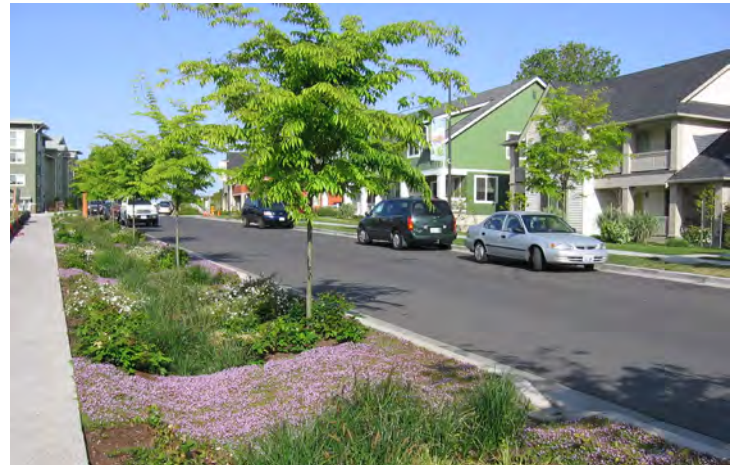
Linear drainage swale
