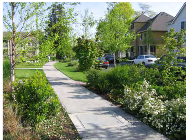
Porous paving on sidewalk
