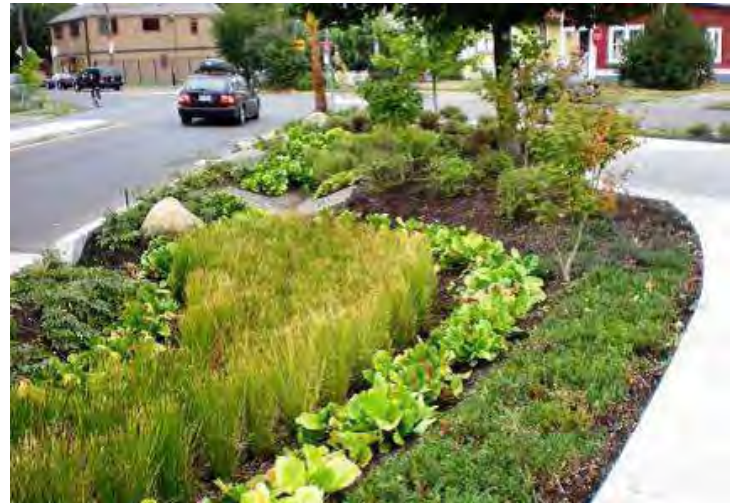
Detention pond integrated with streetscape
