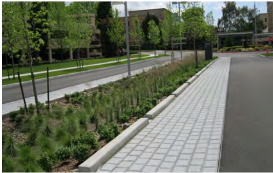
Swale in roadway median with pervious paving
