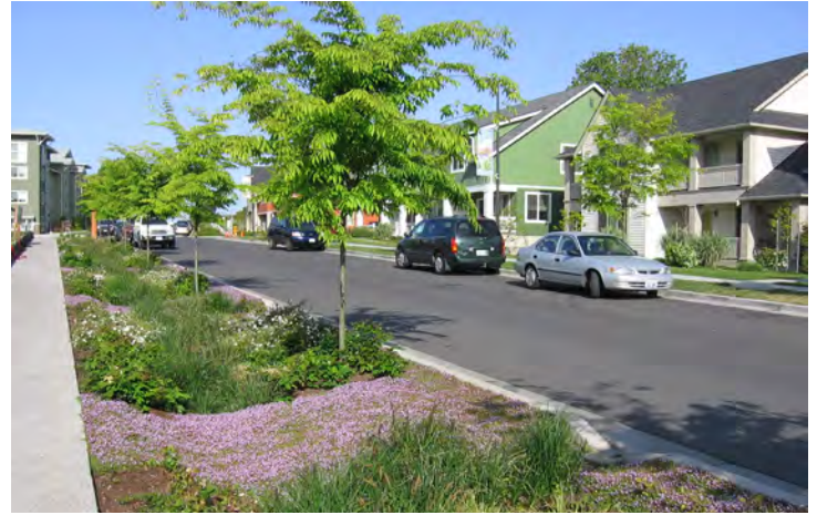
Linear drainage swale
