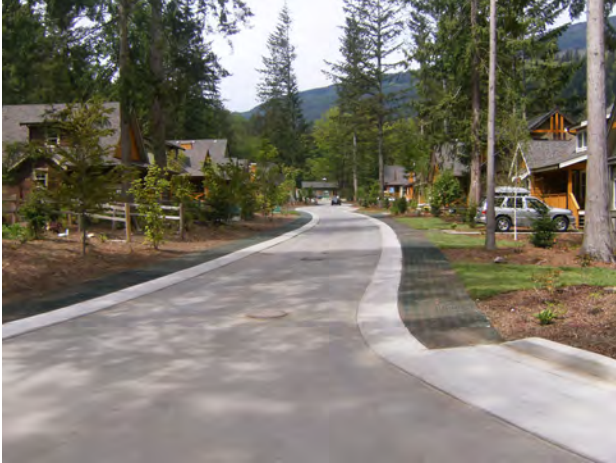
Narrow but functional neighborhood streets
