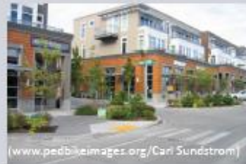
(www.pedbikemages.org/Carl Sundstrom) Curb extensions reduce the pedestrian crossing distance and improve motorists' visibility of pedestrians waiting to cross the street. They can also serve as good locations for bike parking, benches, public art, and other streetscape features.
