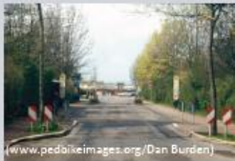
(www.pedbikemages.org/Dan Burden) A "Choker" is a pinch point placed on either side of the street to narrow the center of the lane such that two drivers have difficulty passing through simultaneously. They are appropriate where travel speeds are already low.
