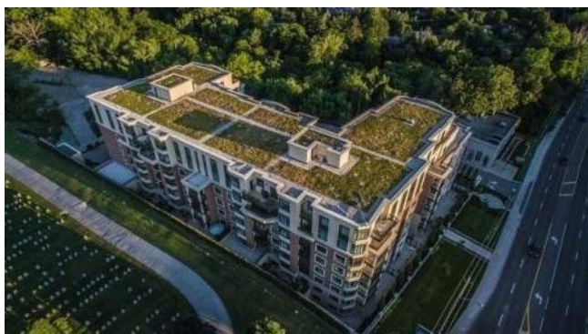
Figure 2 – Green Roof Photo 2
