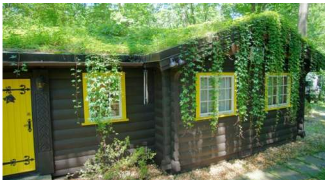
Figure 1 – Green Roof Photo 1
