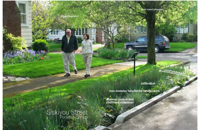
Integrated stormwater treatment
