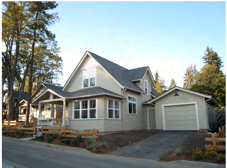
Front porches, generous windows, garage setback
