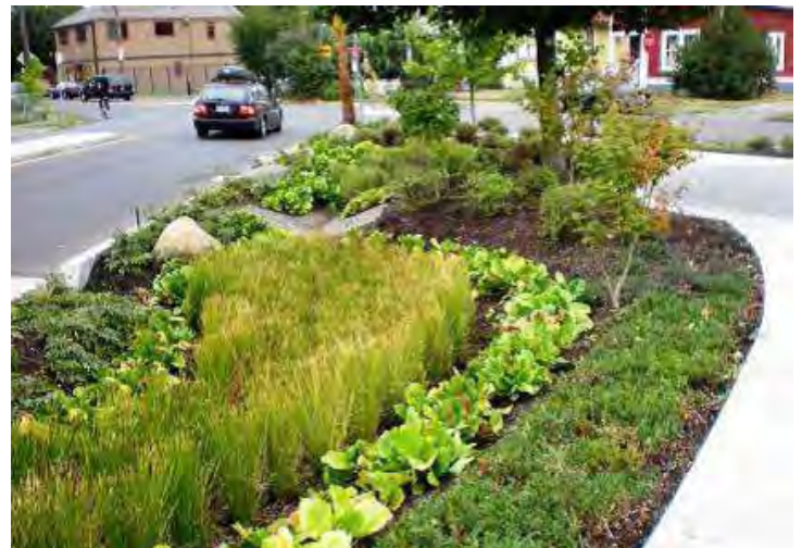
Detention pond integrated with streetscape
