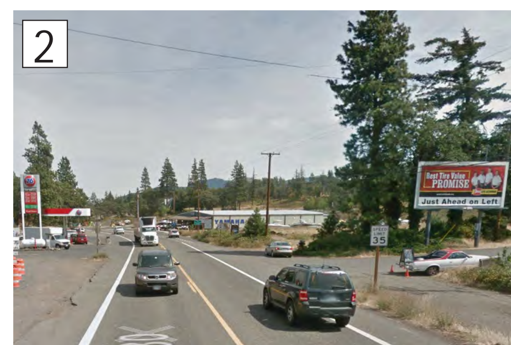
2 Cascade Avenue itself is auto-oriented, with another gas station sign, a billboard and no pedestrian or bicycle facilities. Commercial property frontage is not well-defined.
