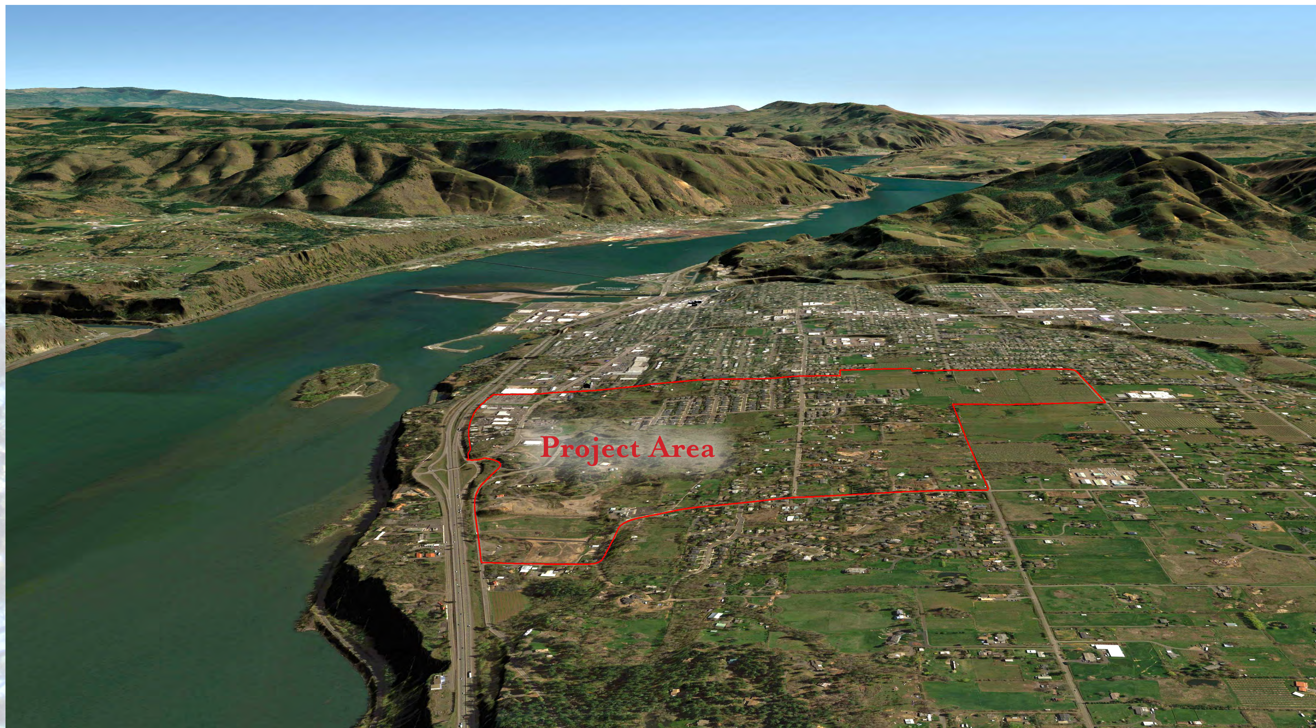
View of Project Area and Columbia River Gorge, looking East
