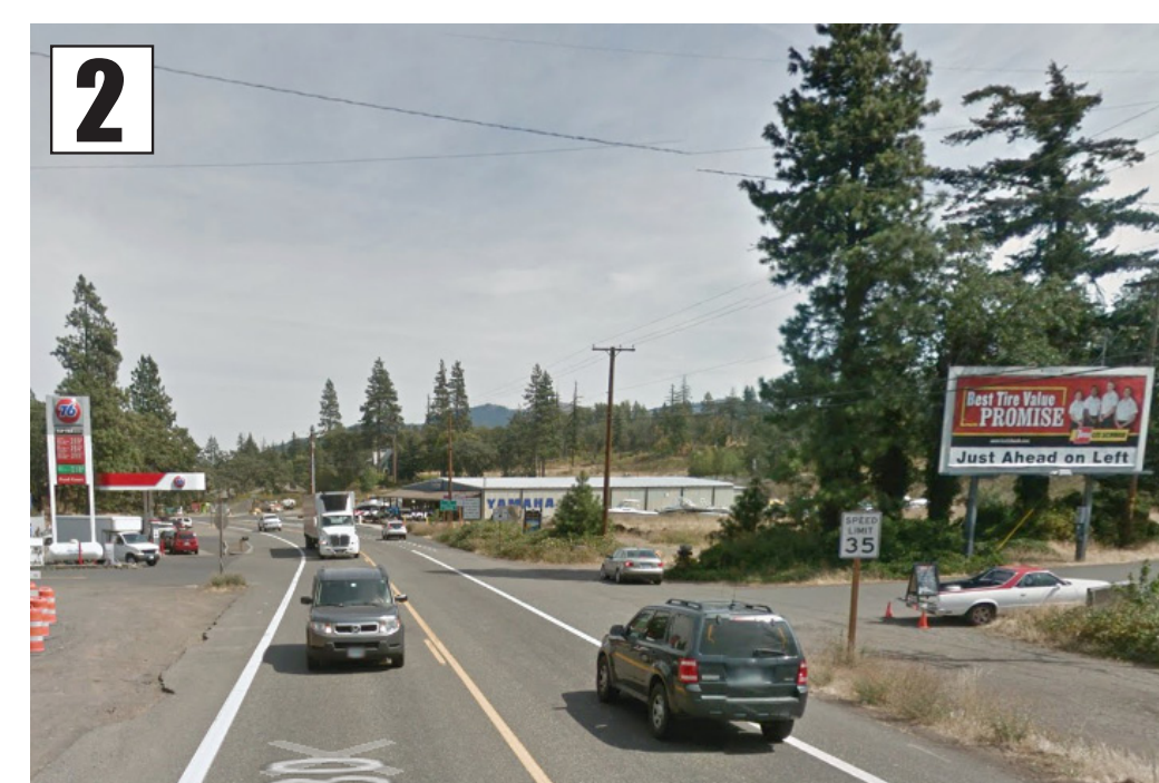
2 Cascade Avenue itself is auto-oriented, with another gas station sign, a billboard and no pedestrian or bicycle facilities. Commercial property frontage is not well-defined.
