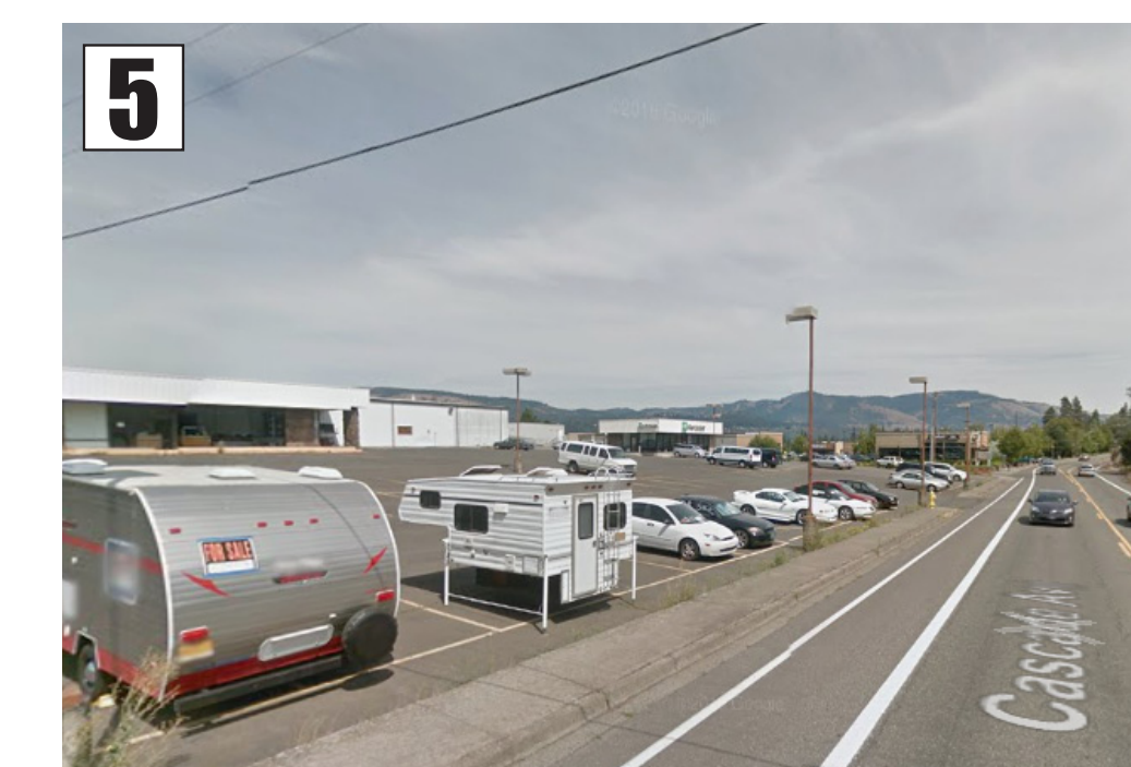
5 Cascade Avenue has intermittent sidewalks and unscreened parking lots, making the district feel automobile-dominated.
